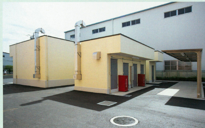
危険物倉庫(1,2,3,5,6類)
